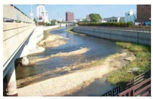
**Figure 2.71** *MINIMALLY ACCEPTABLE shoaling within a concrete lined channel. (MN)*
