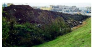
**Figure 2.10** *UNACCEPTABLE, unapproved encroachment. Material stockpiled against the levee. (OK)*
