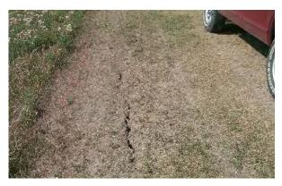
**Figure 2.33** ACCEPTABLE cracking in clay levee with shrinkage cracking caused by dry conditions. (MN)
