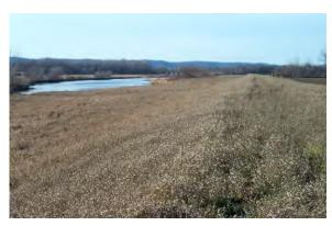
**Figure 2.30** UNACCEPTABLE levee with knee-high grass, making visual inspection nearly impossible. (MN)
