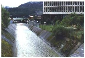
**Figure 2.74** *ACCEPTABLE concrete lined channel.* (AK)
