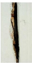
Figure 2.46 Detail of the crack in Figure 2.45, showing the exposed rebar that tied the two monoliths together. (MN)
