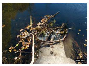
**Figure 2.22** Beavers attempting to block the culvert passing through a gated embankment. (MN)
