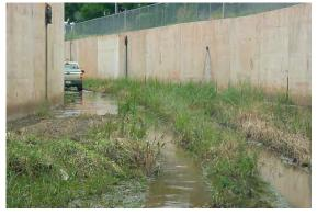
**Figure 2.75** *UNACCEPTABLE vegetation and extensive sediment in channel. (TX)*
