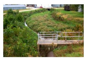
**Figure 2.56** UNACCEPTABLE vegetation and sediment in interior drainage channel. (IA)
