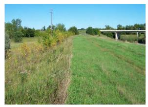
the root ball removed, the voids filled **Figure 2.32** UNACCEPTABLE long grasses and with impervious material and the fill trees on levee side slopes. (ND)
