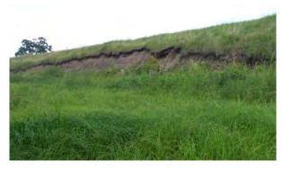
Figure 2.17 UNACCEPTABLE earthen embankment failure.~(MN)
