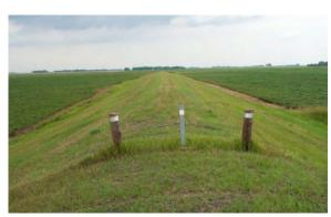
**Figure 2.5** MINIMALLY ACCEPTABLE. Field encroaches on levee easement. The landowner has tilled the soil right to toe of the levee, and was requested to stay back at least 10 feet. (ND)
