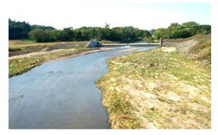
**Figure 2.70** UNACCEPTABLE channel shoaling below a control structure. The original channel bottom extended all the way to the riprapped banks. There is an estimated 2-3 feet of sediment in the channel, mostly from upstream field erosion and highway construction. (MN)
