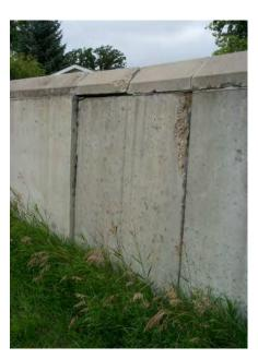
Figure 2.49 UNACCEPTABLE monolith movement in floodwall. The monolith shown in the photo has tilted about 6 inches riverward as well a vertically. Note the movement when compared to the adjoining monolith and the top cap. As the monolith moved considerable spalling has occurred along the joint. This project is monitored very closely during flood events. (ND)
