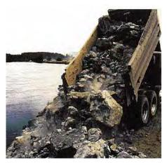
**Figure D.10** Placement of Riprap. Careful use of an excavator may allow for more accurate placement than is shown above.
