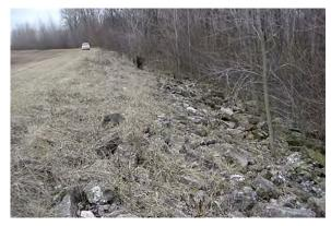
**Figure 2.28** *UNACCEPTABLE. Tree and sapling growth is well established within the riprap protection on an earthen levee. This overgrowth must be removed. (MO)*
