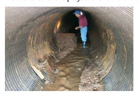
Figure 2.61 UNACCEPTABLE, Failing corrugated metal pipe. DO NOT WALK INTO A FAILING CULVERT LIKE THIS. This section has actually separated, allowing the surrounding soil to enter the pipe and the overburden to collapse. This sponsor was denied rehabilitation assistance due to this maintenance deficiency.
