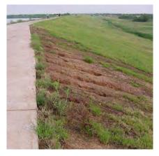
**Figure 2.1** *UNACCEPTABLE erosion of levee slope. (TX)*
