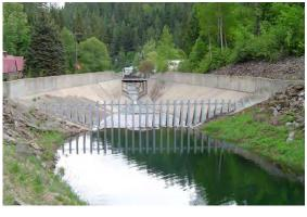
**Figure 2.73** ACCEPTABLE intake structure upstream of the concrete channel. (ID)
