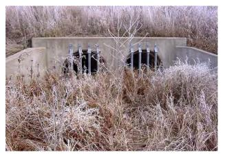
Figure 2.60 MINIMALLY ACCEPTABLE. vegetation blocking the concrete culvert must be removed. (KS)
