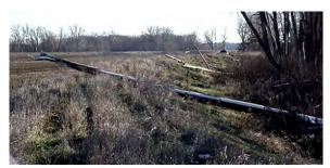
**Figure 2.9** UNACCEPTABLE encroachments on earthen levee. Fallen woody debris requires removal. (KS)
