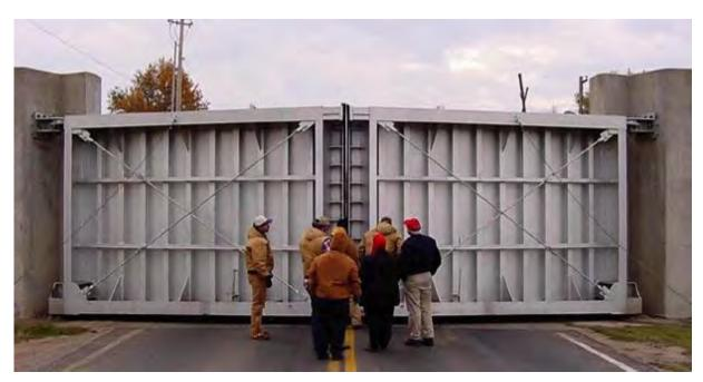
Figure 2.42 ACCEPTABLE floodgate in a levee. (KS)
