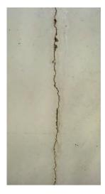
**Figure 2.43** MINIMALLY ACCEPTABLE 1/8<sup>th</sup> inch crack extends through concrete floodwall and needs to be sealed to prevent further damage. (MN)
