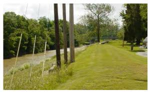
**Figure 2.7** UNACCEPTABLE levee encroachments. Utility poles in levee embankment. (IN)
