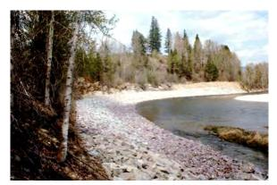
**Figure 2.25** ACCEPTABLE riprap for erosion control. (MT)
