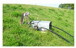
**Figure 2.8** UNACCEPTABLE encroachment. Piping for lawn irrigation system drilled through levee without approval. (ND)
