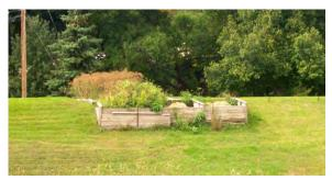
**Figure 2.13** *UNACCEPTABLE encroachment. Gardens and compost bins located on levee crest and riverward slope.* (ND)
