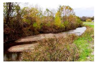
Figure 2.69 UNACCEPTABLE vegetation in channel and sediment shoaling. (OK)
