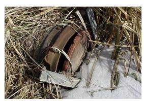
**Figure 2.66** UNACCEPTABLE flap gate in earthen levee. (Broken hinge and vegetation growth.) (MO)
