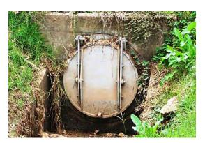
**Figure 2.65** *UNACCEPTABLE vegetation* around flap gates in earthen levee. (OK)
