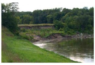
Figure 2.15 UNACCEPTABLE. Slope failure and Figure 2.16 UNACCEPTABLE. Slope failure and erosion caused by inadequate channel bottom and erosion on a channel improvement project. (MN) side slope protection. This was a direct result of bottom scouring that undercut the levee slope and erosion caused by turbulent flow at the end of the bank protection. (ND)
