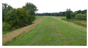
**Figure 2.31** UNACCEPTABLE. Levee is mowed but trees and longer grasses within levee easement area. Trees are greater than 2" in diameter. (MN)
