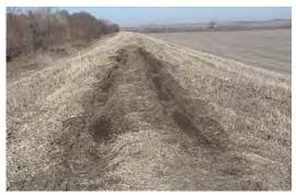
**Figure 2.37** UNACCEPTABLE ruts in levee crown require fill. (MO)
