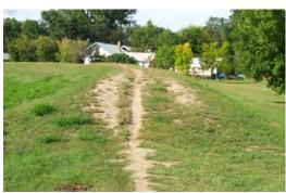
**Figure 2.36** MINIMALLY ACCEPTABLE levee rutting caused by pedestrian and bicycle traffic. (ND)
