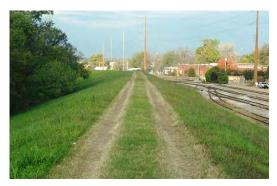
**Figure 2.39** *UNACCEPTABLE rutting in levee.* (OK)
