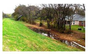
**Figure 2.53** *UNACCEPTABLE interior drainage* at the toe of an earthen levee. (OK)
