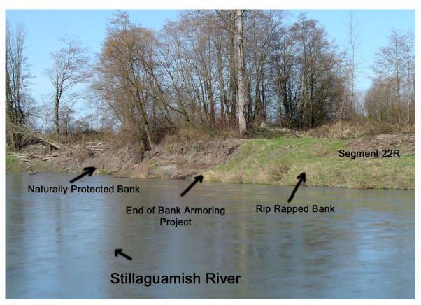
**Figure 2.23** Flood damage on a naturally protected bank, as compared to damage on an adjacent bank which was protected with riprap. (Note that even though the riprap clearly protected the area during the flood, if it was observed an inspection it would have probably been rated Minimally Acceptable because the grass would have prevented an inspector from properly examining the riprap.) (WA)
