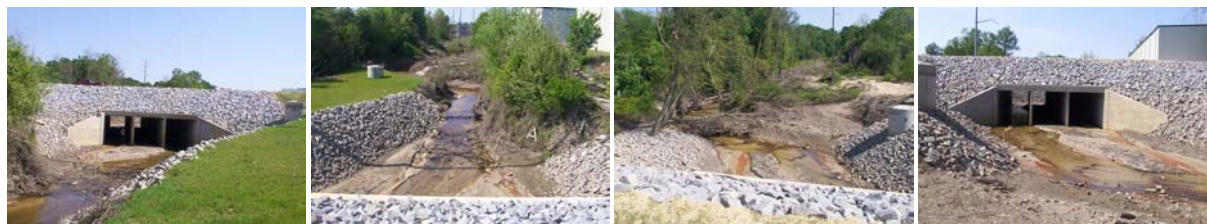
Figure 18. Examples of Culvert Photographs
