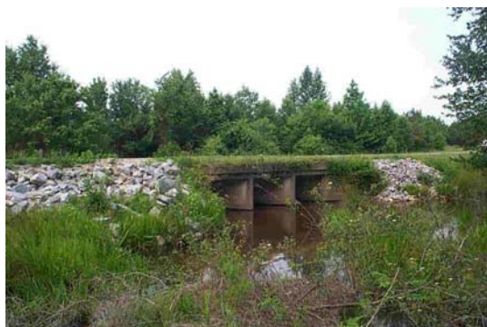
Figure 48. Example of Approximate Survey Photograph
