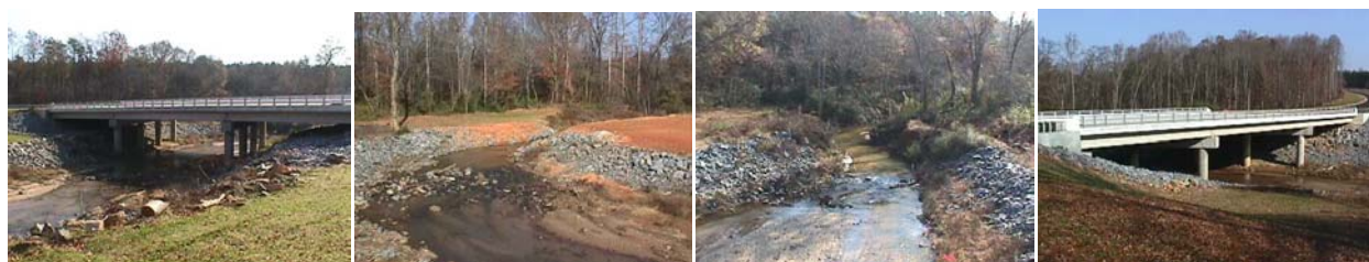
Figure 6. Examples of Bridge Photographs
